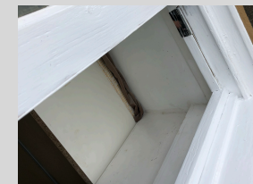
We router our draught strips into the sash.
